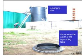
Fig. 5. Throw away the cover of the repumping tank after explosion
