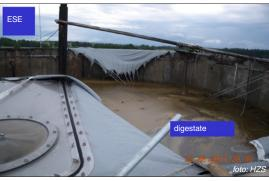
Fig. 6. View into the damaged inner tank of fermenter, which is located in the protective area of ESE
